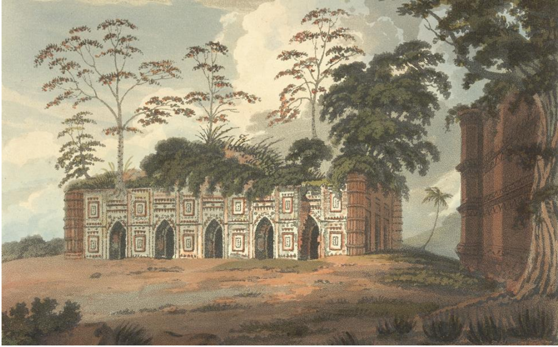
Figure 18 Architectural heritage of Maldah – Multi domed, rectangular Tanteepara Masjid, Gaur. Source: http://www.bl.uk/onlinegallery/onlineex/apac/other/largeimage68598.html
